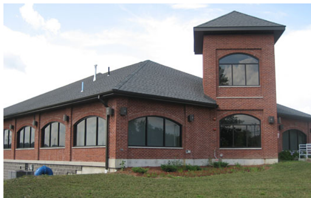
The Harold P. Naughton Water Filtration Facility
